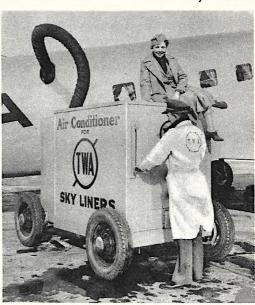
Cooling the plane's interior in the summer and heating it in winter just before it starts out on its trip across the skies is the duty of this four-wheeled electric air conditioner.
